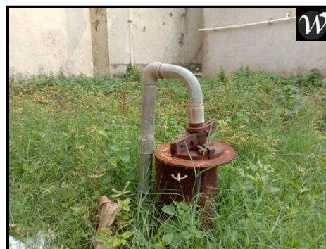
Figure 4. Bore well system in college campus
